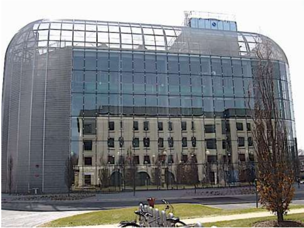
Figura 50. University of Chicago South Campus Chiller Plant (Burimi): angwe23, 2009. (Flickr). Creative Commons–NoDerivs 2.0 Generic
