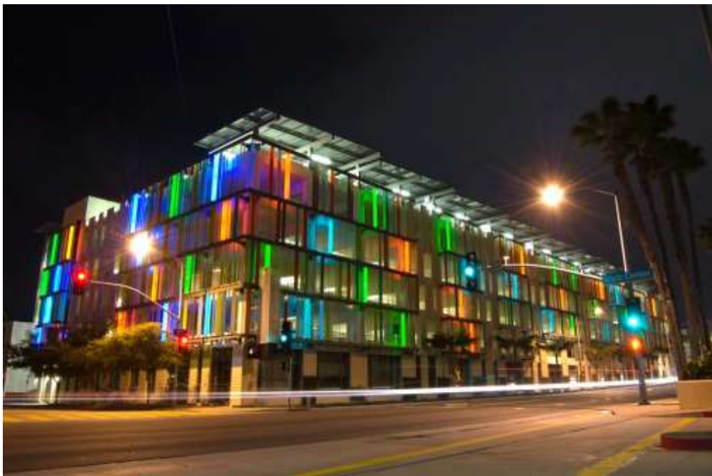
Figura 183. Parking Garage, Santa Monica LEED Parking
