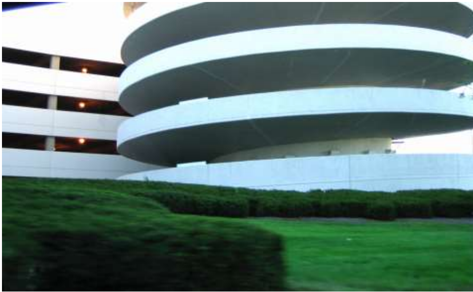
Figura 190. Parking garage ramp Indianapolis IN airport (Burimi): jill, 2005. E licensuar nga Creative Commons Attribution ShareAlike 2.0 Generic
